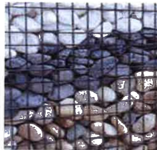
11 Gabion Feature Wall Finish or Similar
