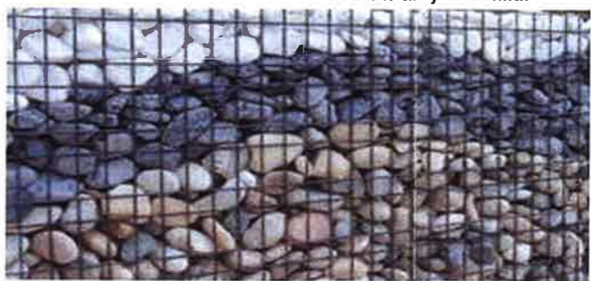
11 Gabion Feature Wall Finish or Similar
