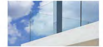
04 Clear Balustrade Glazing
