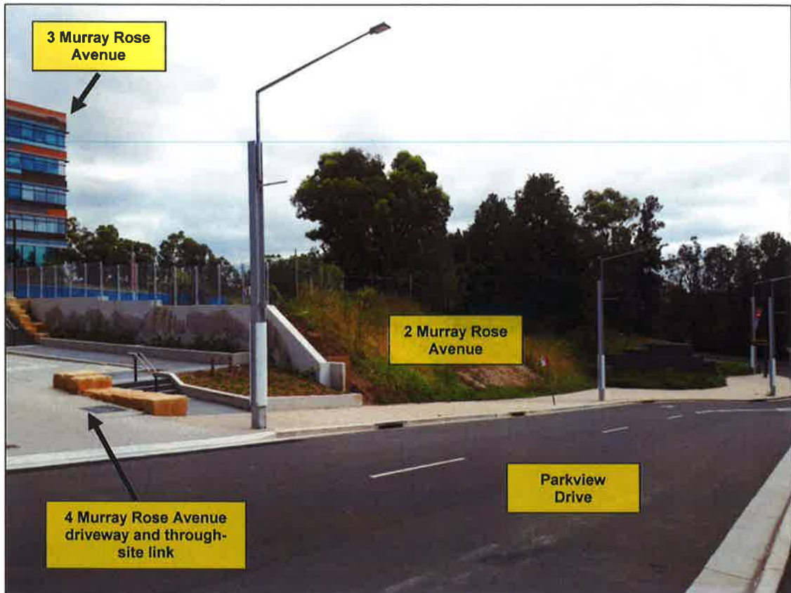
Figure 8 | 2 Murray Rose Avenue viewed from Parkview Drive looking north-east (Base source: Department's photograph)
