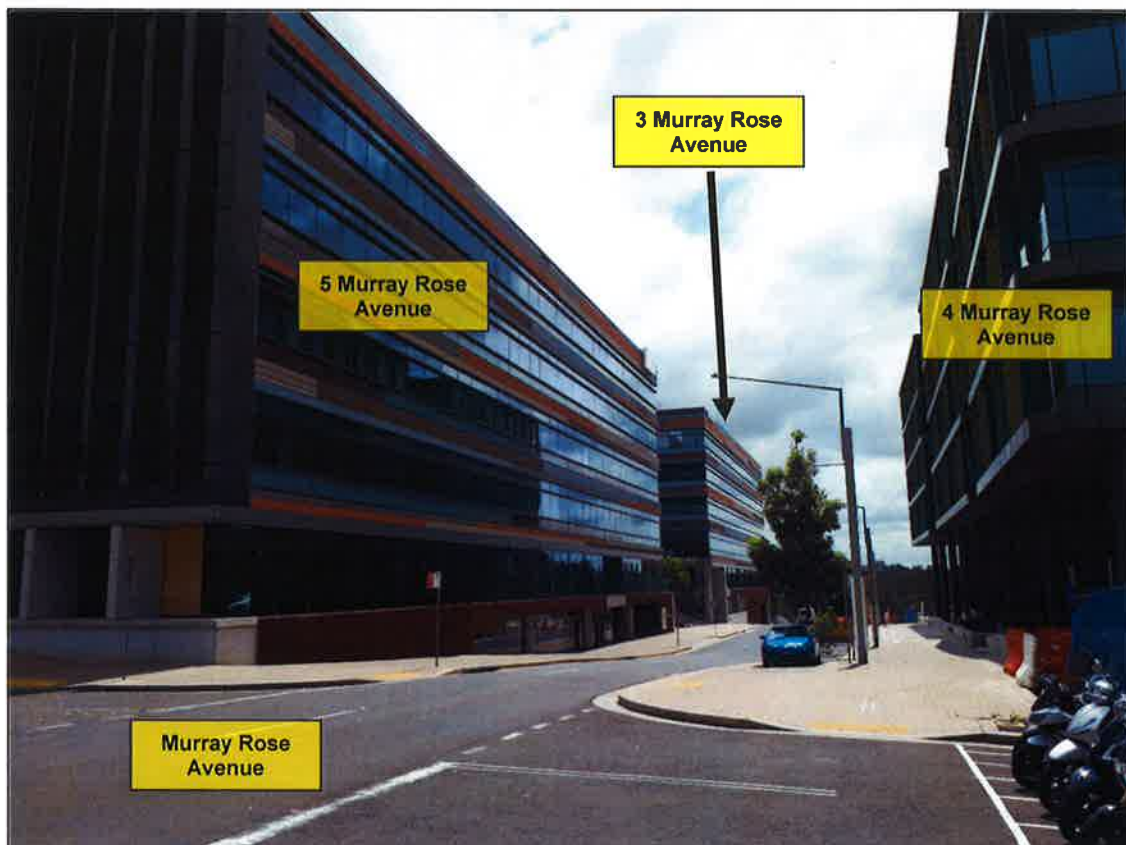
Figure 9 | 3, 4 and 5 Murray Rose Avenue viewed from Murray Rose Avenue looking east (Base source: Department's photograph)
